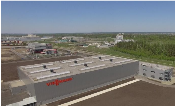
Viessmann, Lipetsk/ Russia New construction production, logistics, office
