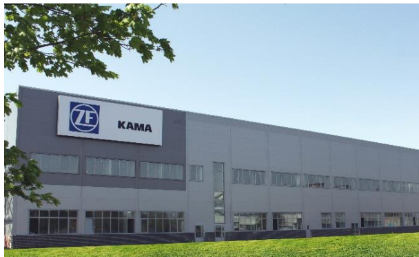
ZF Kama, Naberezhnye Chelny/ Russia New construction (Brownfield) gearbox production
